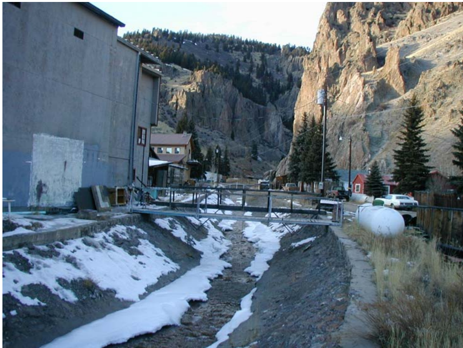
Figure 1: Willow Creek at Creede flume, looking upstream. At station 09+25.
