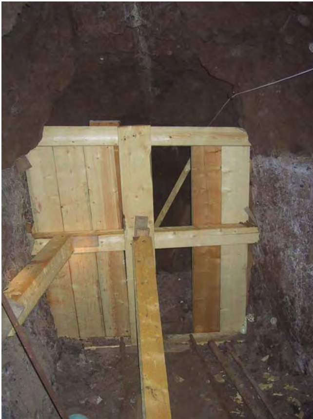
Figure 8. Partially Completed Bulkhead
