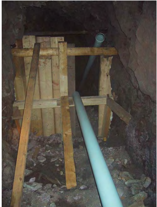
Figure 9. Bulkhead and Piping
