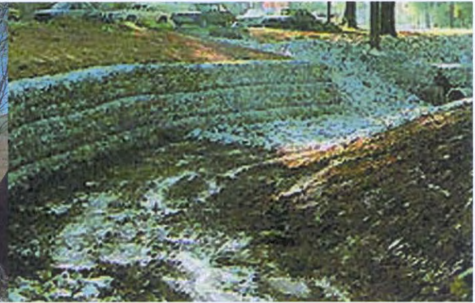
using gabions for remediation of river bed
