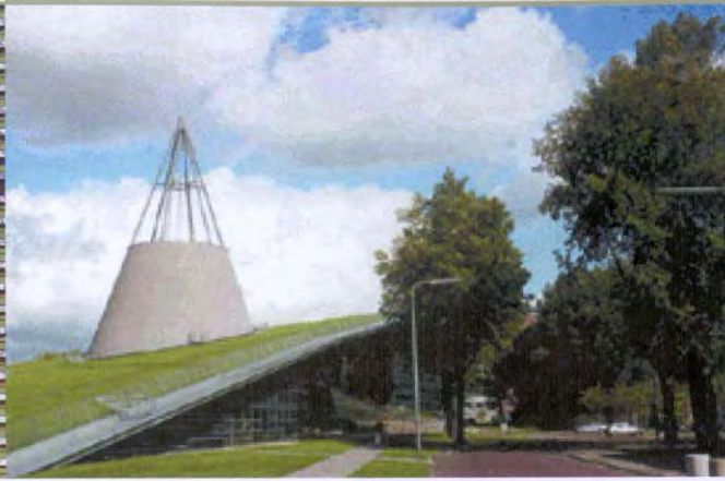
roof as landscape - good for insulation and acoustics library, delft, mecano architects
